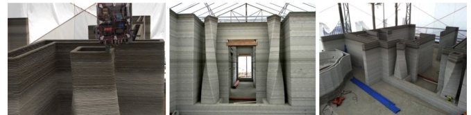
Figure 19: The interior structure of the hotel with 3D printing in Philippines [63]
