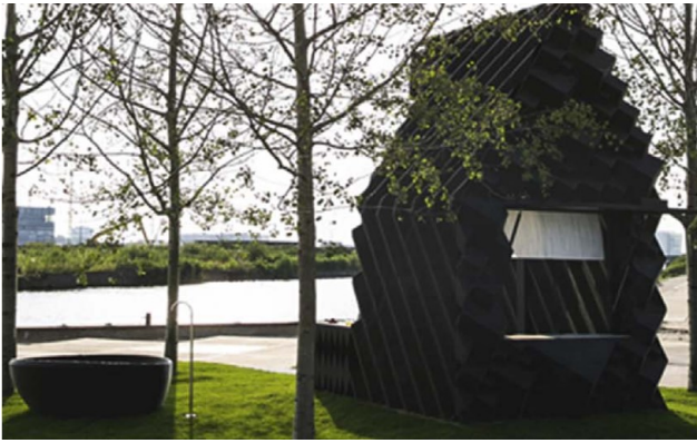
Figure 17: 3D printed house by Dus Architects [61]
