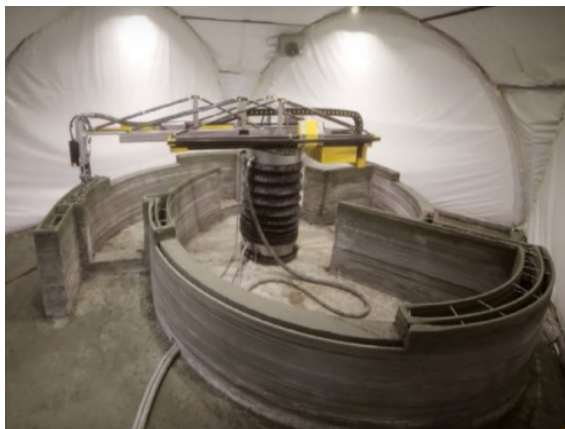
Figure 12: Advanced 3D printing robotic model (Articulated type)
