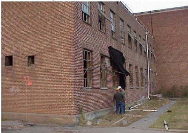
Fig. 12. Façade of the building and blast chamber showing solid Wall #2 (on the left) and Wall #3 with windows on the right (Zapata J. B. and Weggel C. D., 2008)
