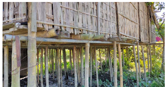
Fig 1: Stilts of the superstructure
