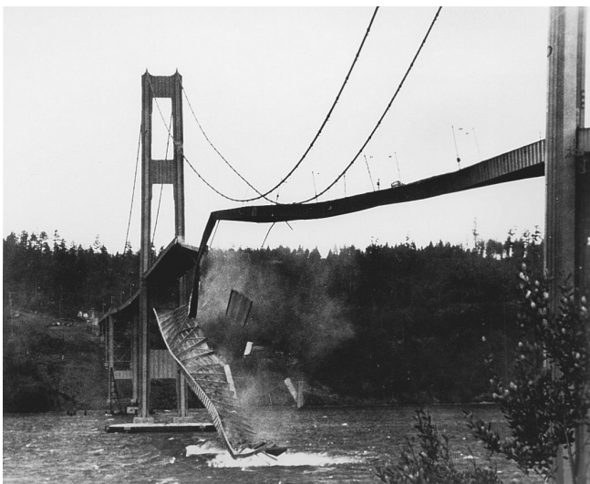
Fig.2 Failure of Tacoma Narrow Bridge
