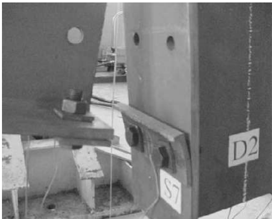
Fig. 3. Failure of connection
